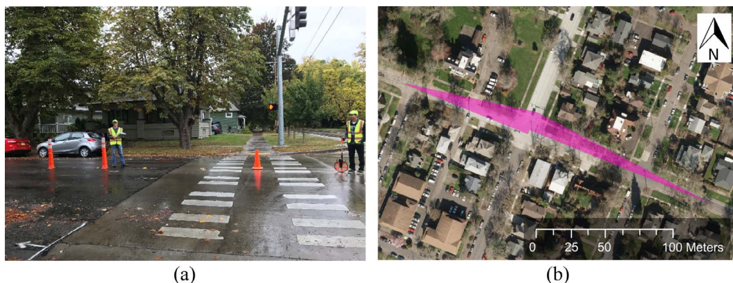
Fig. 8. Southbound approach SSD triangles of intersection of SW Jefferson Way and SW 9th: (a) SSD study in progress and (b) SSD triangles overlain on Arcmap image.
