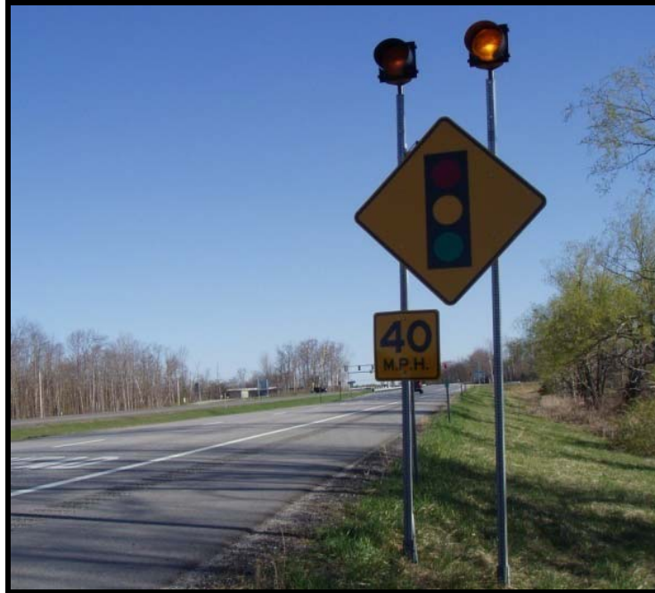
Figure 11 Typical Advanced Warning Flasher (AWF)
