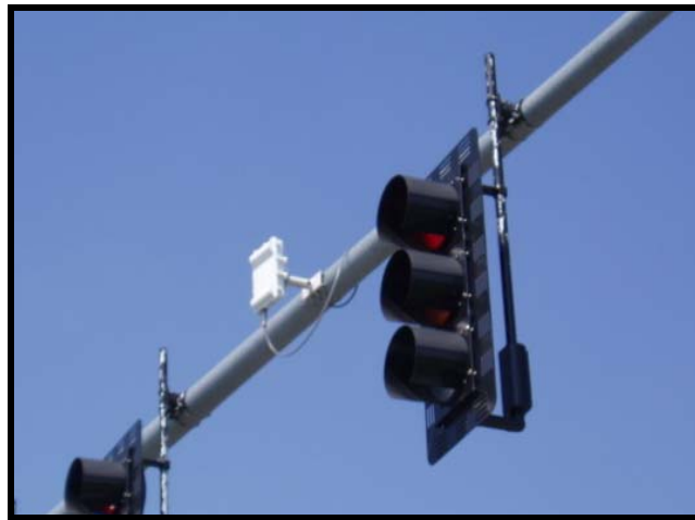
Figure 26 Installation of the SmartSensor in Vermont
