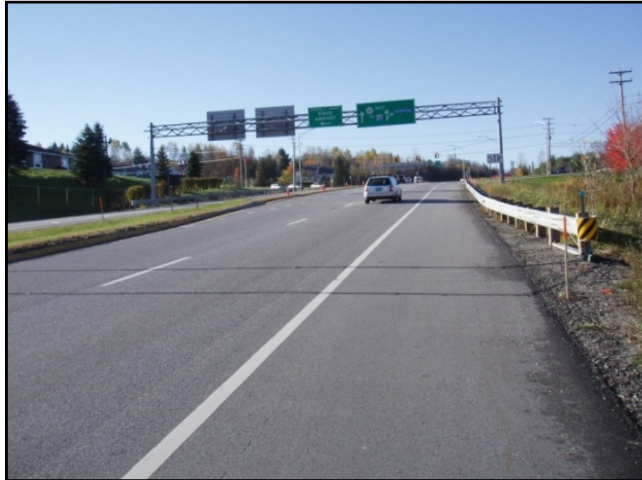
Figure 12 Example of Typical ATR Installation
