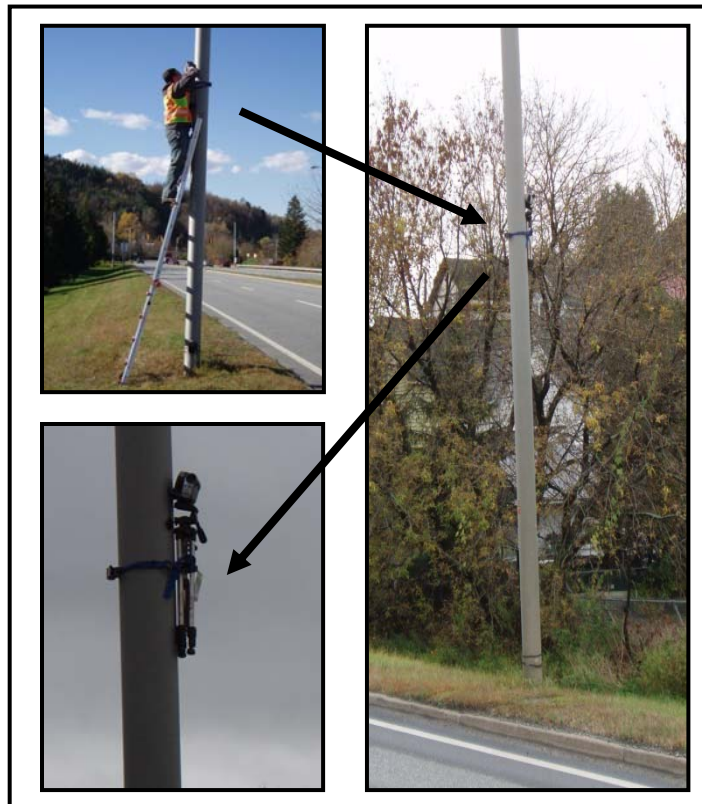
Figure 13 Example of Typical Video Camera Installation
