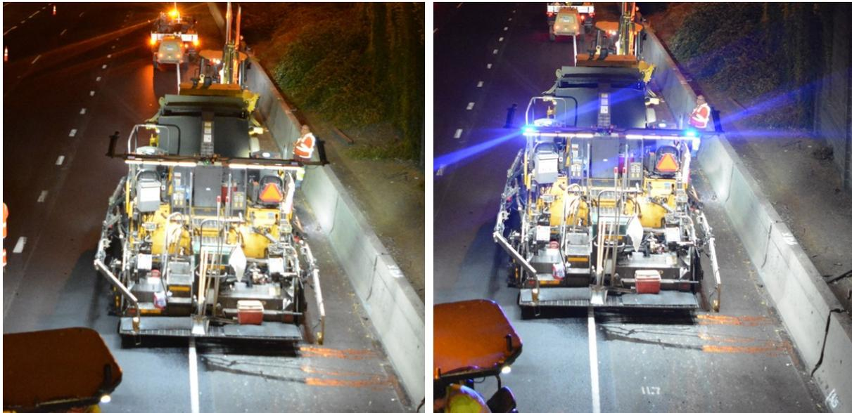
**Figure 4.1: Paver with flashing blue lights off (left) and blue lights on (right)**
