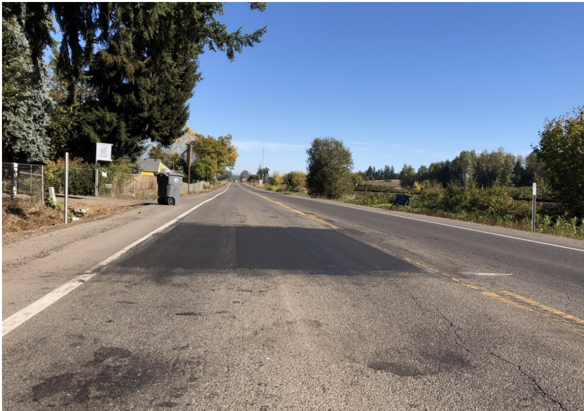
Figure 3.3: After condition: Paved TRS at far location
