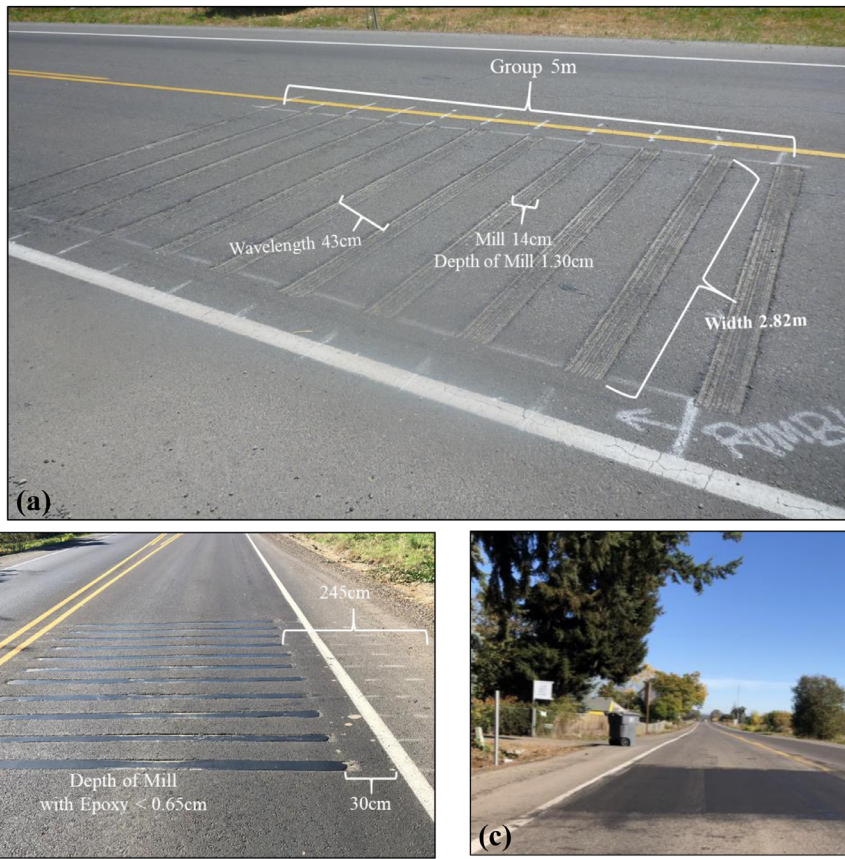
Fig. 3. (a) Before condition: TRS geometric characteristics. (b) After condition: epoxy filled TRS at near location. (c) After condition: paved TRS at far location.
